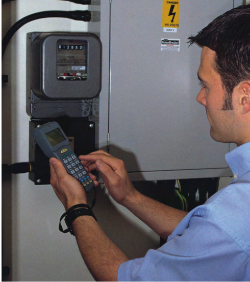
Entering readings directly into the handheld reduces data transcription errors and speeds up billing tasks.
